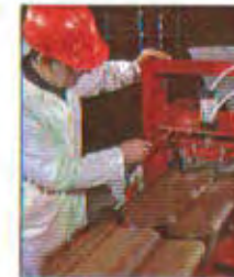
Wet tiles cut to length
